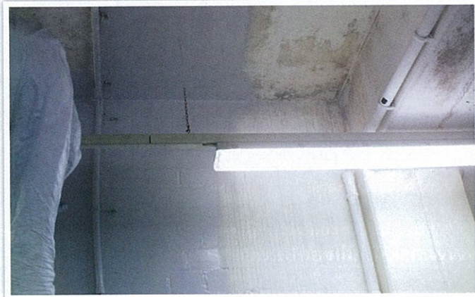
A primer applied onto surface seals old biomass
