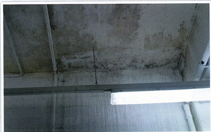
Sanitization of surface is not sufficient as disinfectants cannot reach deeper layers of material
